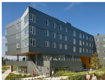
Bellevue College, Bellevue, Wash. (Photo courtesy of NAC Architecture)
