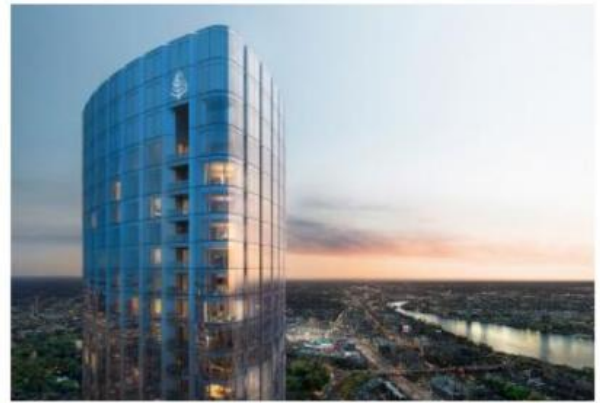
The building envelope of the 61-story Four Seasons Hotel and Private Residences at 1 Dalton St. in Back Bay is primarily glass. An argon gas filled air space combined with metallic coatings produces a high shading coefficient and an energy-efficient insulating value.
